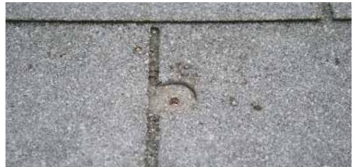
7. Eject the cut out ring of the asphalt shingle from the tool and/or pick the debris out of the produced counter bore
