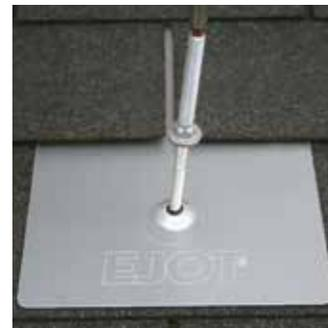
13. The Solar Fastener has to be installed square to the roof surface. A maximum deviation of about 5° to the roof surface is acceptable.
