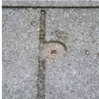
3. When needed, lift roof shingle, right above placement of the fastening position, with roofing bar, to allow the flashing to be shifted in the correct mounting position.
