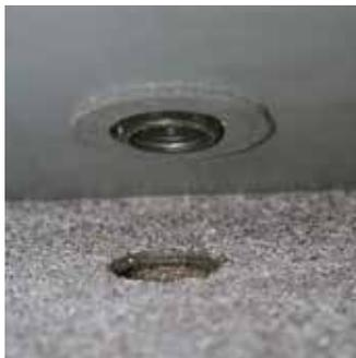
12. Insert the EJOT Fastener through the lined up Flashing and pilot hole in the rafter while using a drilling machine and a rotation speed of about 450 - 500 Rpm.
