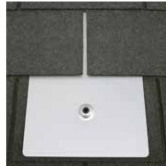
11. Line up pilot hole in the rafter with EJOT Flashing hole and make sure, that the sealing element is fitted in the countersunk hole of the shingle.
