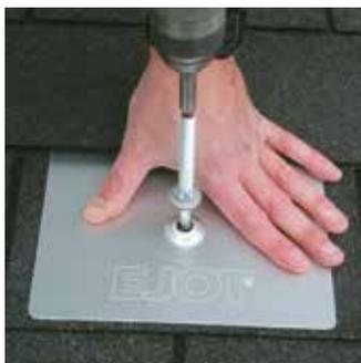
14. Tighten the fastening element while reviewing the EPDM compression of the sealing ring.
